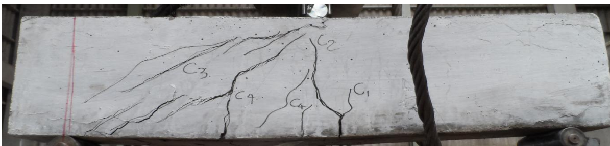
6.1 Failure Pattern of BR4MPΦ30
