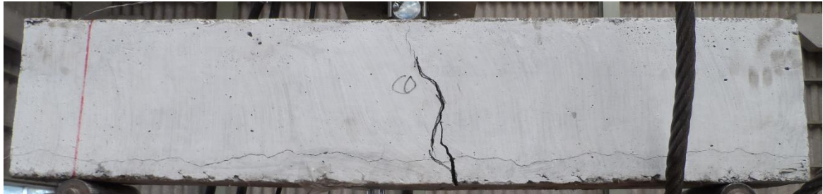
6.5 Failure Pattern of BR4MPΦ25
