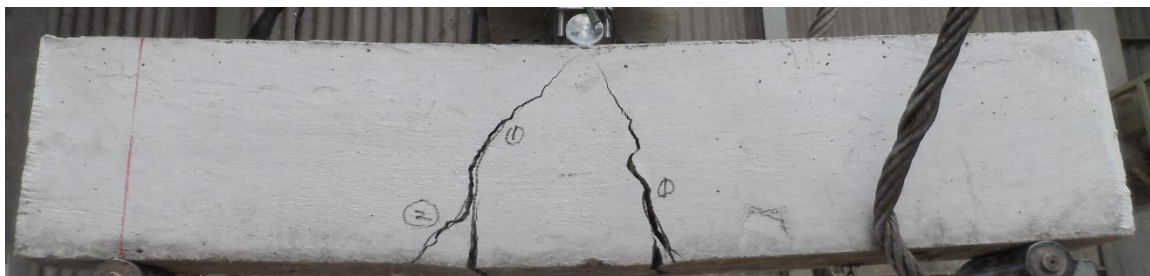
Figure 7: Failure Pattern of BR4SBΦ10 (Control Beam)
