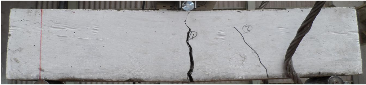
6.3 Failure Pattern of BR4MPΦ20
