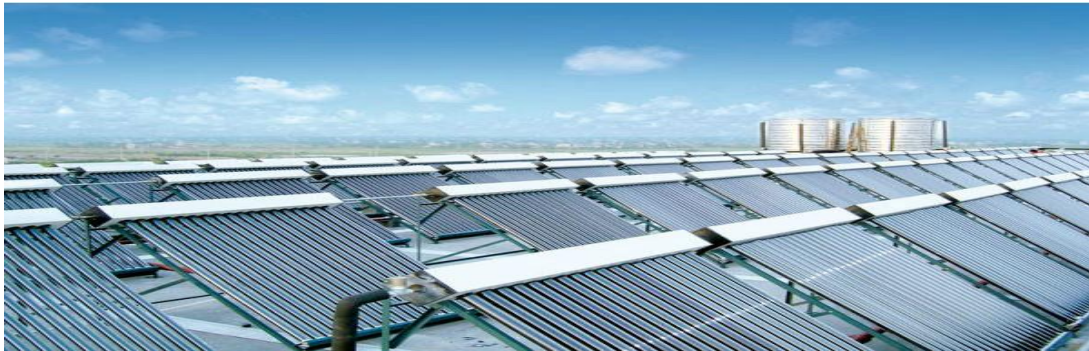
Fig3. shows Solar Water Heating system
